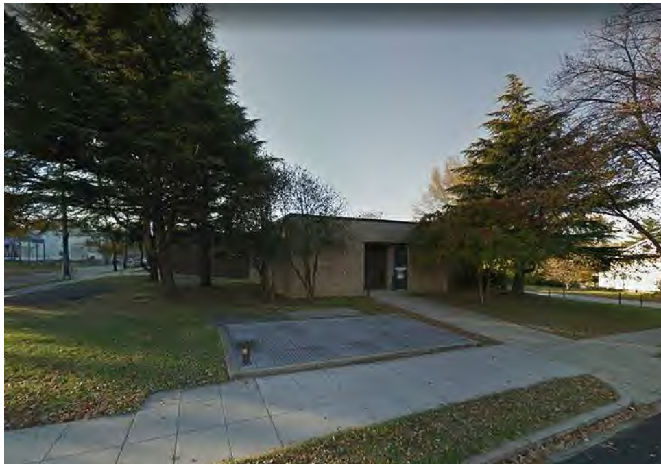
4. ELLICOTT ST WMATA FACILITY
