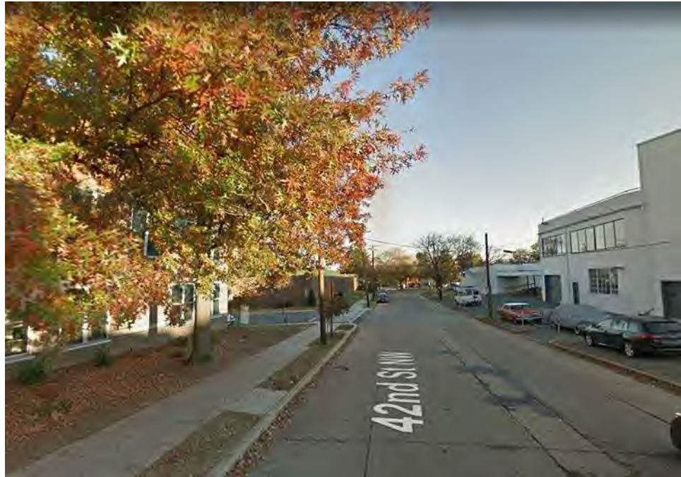
1. 42ND ST LOOKING NORTH
